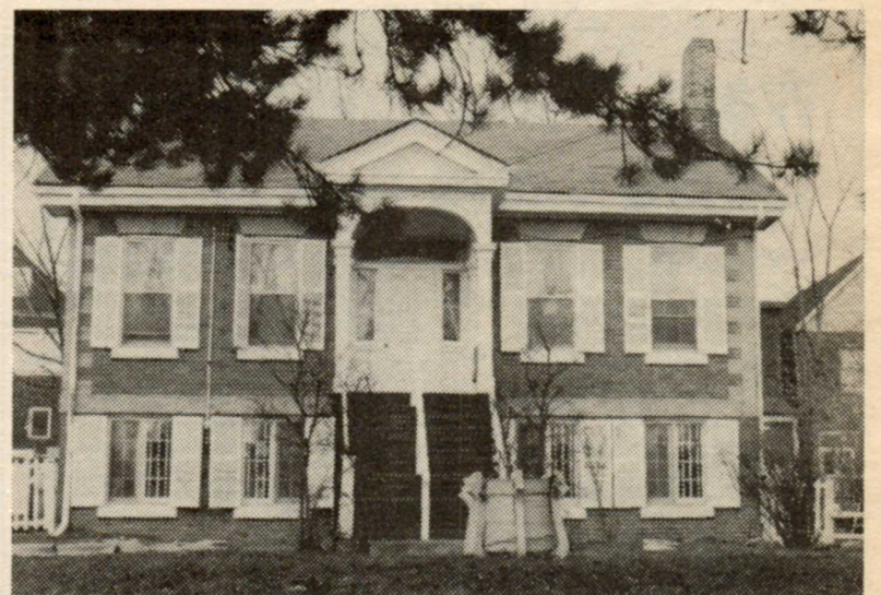
14 Dingwall Avenue. This is a farmhouse (built in the 1850s) of cottage form, and displays typically Georgian features. It has a Georgian door, centre hall plan, large shuttered windows with 6-pane, double-hung sashes, quoins, side-chimney and small verandah (portico).
