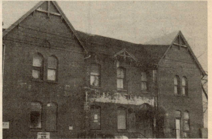
Before and after shots of the Trinity Medical School (1871) on Spruce Street. The beautiful Victorian brickwork pattern has since been covered up with paint. The building cries out for restoration. The first photo is from the Trinity College Convocation Bulletin, Vol. 10, No. 5 — Summer 1973.
