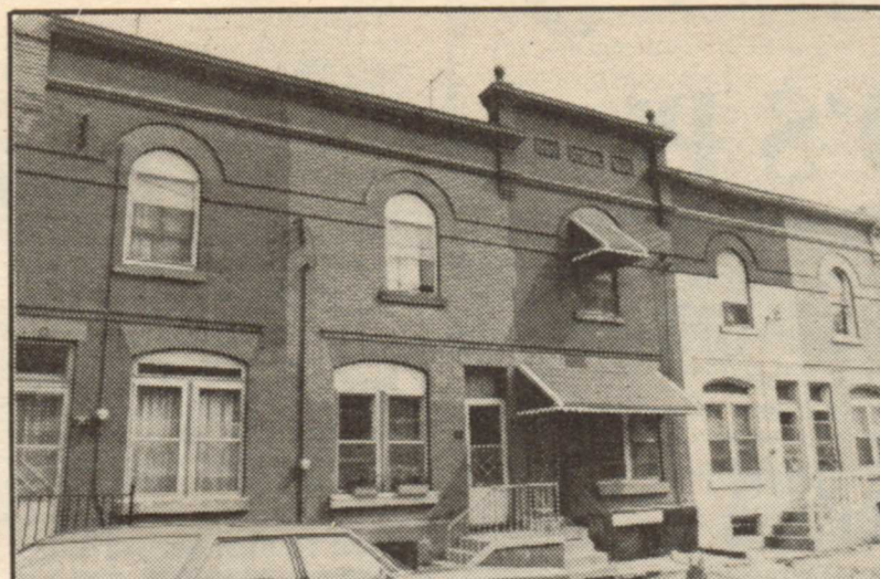
Numbers 18 to 26 Allen Avenue — a set of 1890 brick-fronted houses bearing Romanesque arches in the brick pattern in the second storey. In 1890, this treatment of brick fronts was just beginning to come into fashion.
