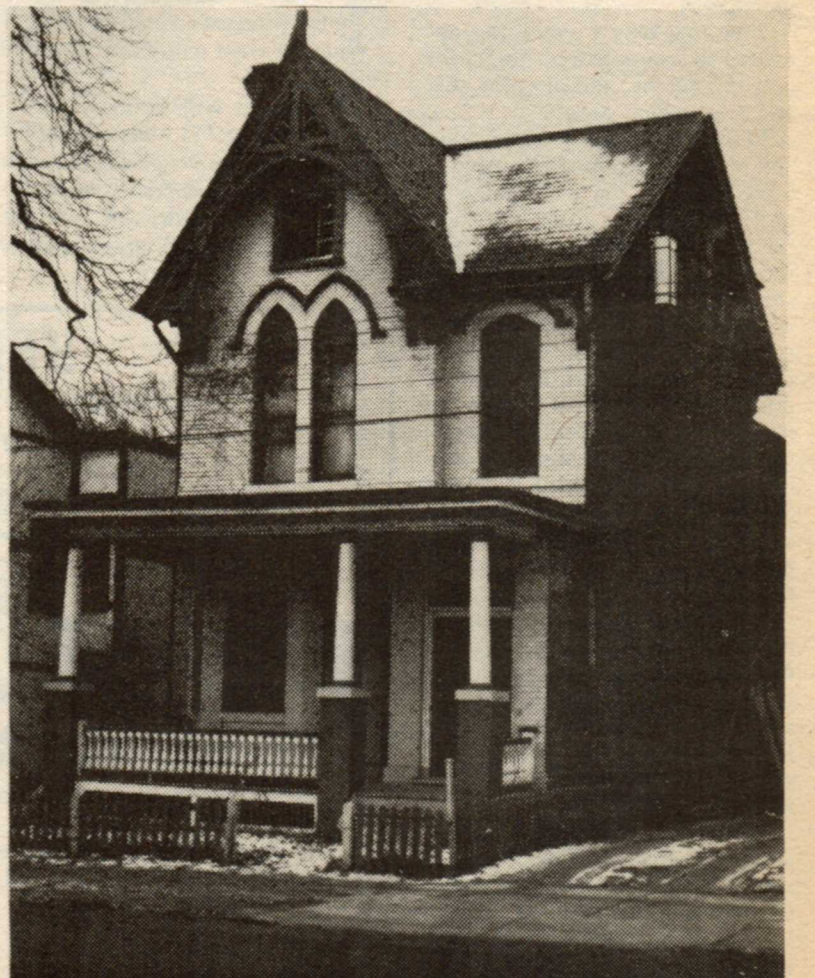
Number 282 Sherbourne street, above, is also considered very historic and is threatened with demolition.
