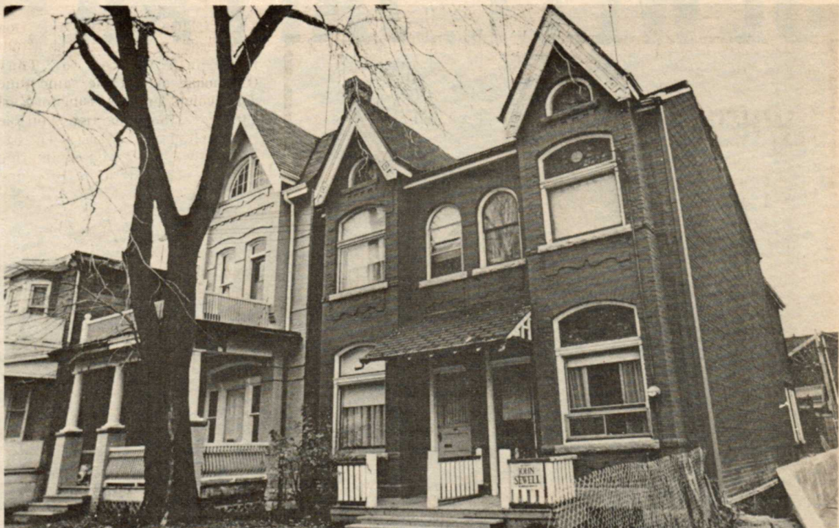
Pictured above are two of the three houses co-operatively owned by Don West Neighbours Group. The houses, located on Ontario street are in the final stages of repair and rehabilitation. The South of Carlton Co-op is hoping to buy five more houses. (Photo by Charlie Dobie)
