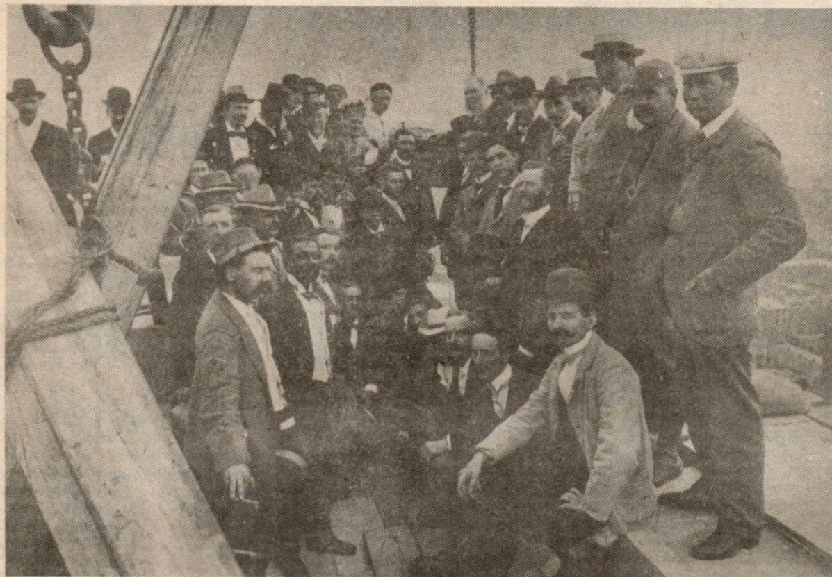
The ceremony of laying the last stone on the tower of the Old City Hall, on July 14, 1898, 245' above the ground. Alderman William Hubbard (Toronto's first black alderman) is second from the left in the foreground. The man with the white sideburns, at the back right centre, is Mayor William Shaw. In the centre is Mrs. Shaw, and to her right — with hat and white bow tie — is E.J. Lennox, architect of this magnificent building. For the complete story on Hubbard, see the George Rust-D'Eye article on page 12. Photo courtesy City of Toronto Archives
