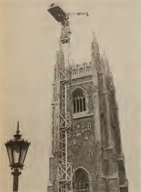
Hart House area was cordoned off for an hour yesterday as this crane hoisted to the top an entire replacement set of bells for the Hart House Tower.
