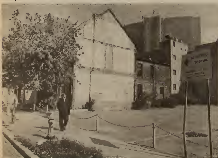
These buildings were scheduled for demolition. Note Hydro building in background.
