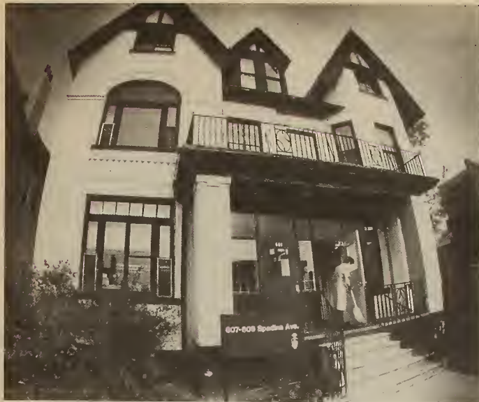
Cleaning continues normally for these two houses, slated for demolition to make way for the athletic complex.
