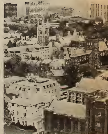
The campus as Campus Centre Project towards stopping the concrete infiltration
