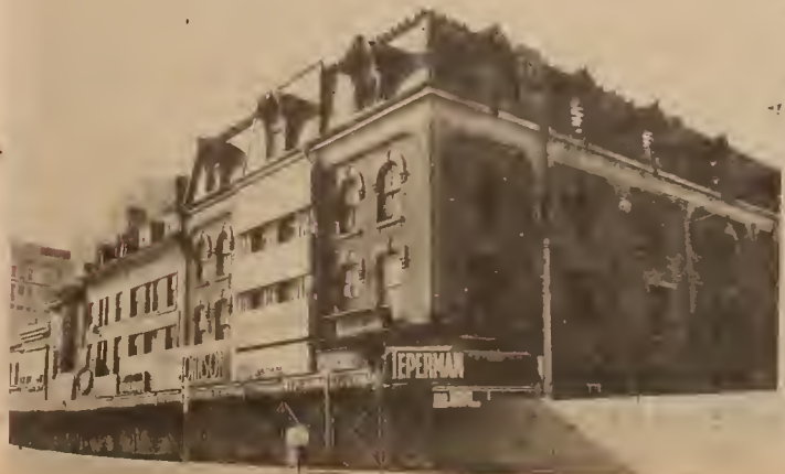
This part of Yonge St. is already under demolition for phase 1 of the Eaton Center plan, which hopes to gobble up three further pieces of land owned by McMaster University. U of T has already sold 188 Yonge to Fairview Corp.
