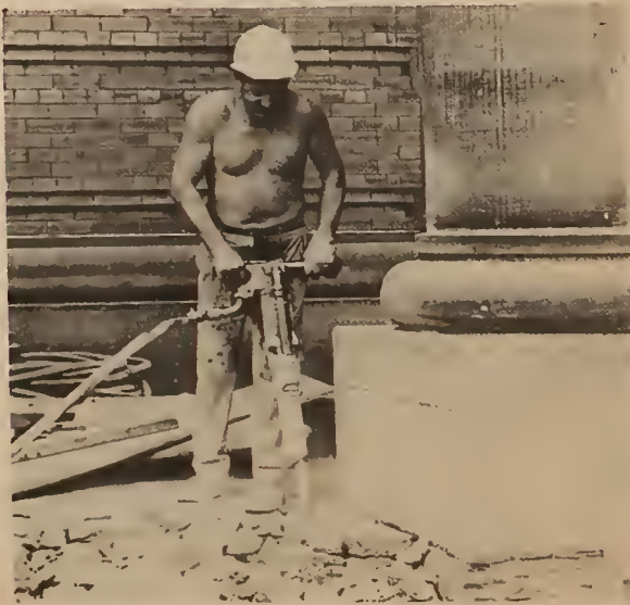
This is a worker busy chipping away at the foundation of our society. Once the mortar is loosened he'll work on the pillars and then he'll be at the gates. But if he suffers a setback he's content with the fact that one of the many programs sponsored by the Unitwit Way can help him and his loved ones.
