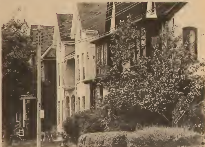
This house above (the one behind the trees) on Sussex Street is owned by U of T and managed by Crown Trust. It has been allowed to deteriorate so much that part of it fell, hitting a tenant.
