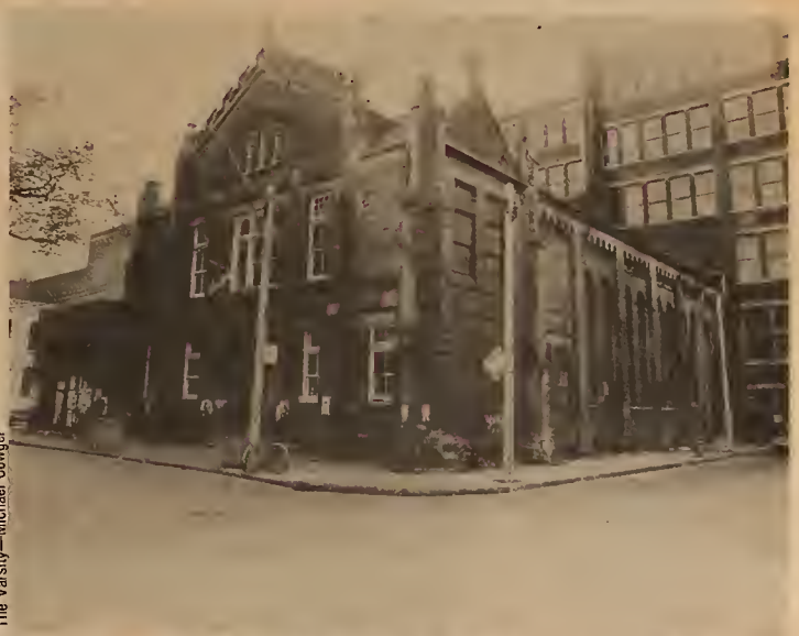
Eaton's applied for a demolition order against this building last week. It is the home of Theatre Passe Muraille, but not for long. Ah yes, the lovely sound of jackhammers.
