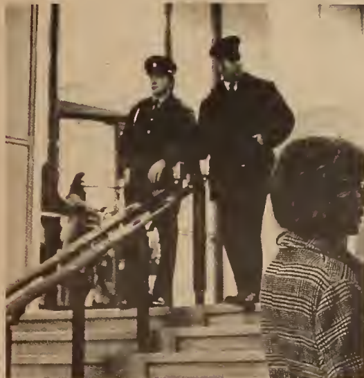
During the demonstration, police guarded main library.
