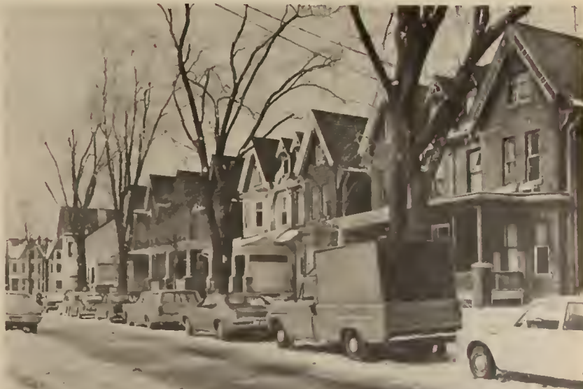
Most homes in the north-west campus will fall to the wrecker's ball as U of T completes expansion.
