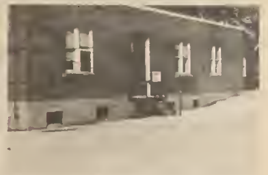
Daycare wants this building, now used as shed.
