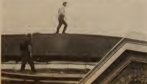
Workmen put last touches on Convocation Hall's new $77,000 roof.
