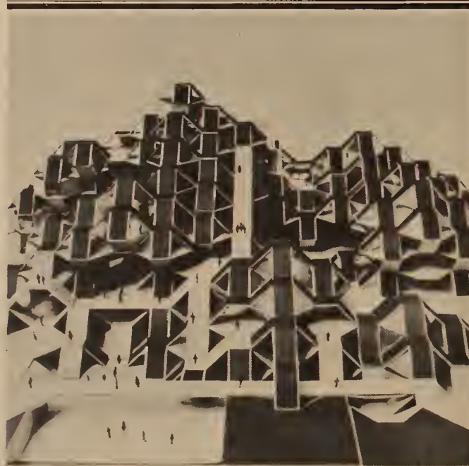
The brilliant but vetoed San Francisco State College Union. A view from the campus green showing the inclined walls forming stairs on the building surface. Dark areas on the other inclined walls represent planting covering and penetrating the structure.
