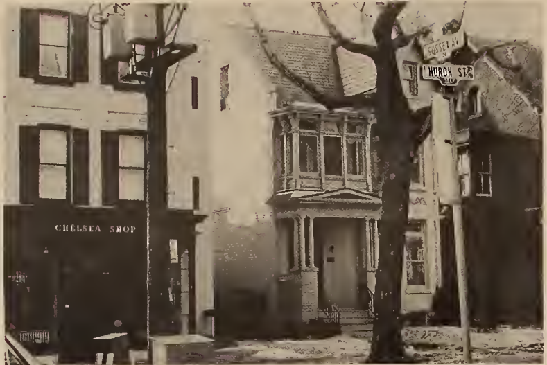
This area is all coming down. What once used to be an expensive residential area will become part of a new university face.
