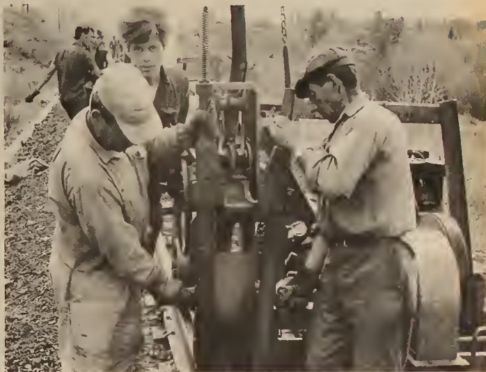
Pulling spikes on northern railway repair gang.
