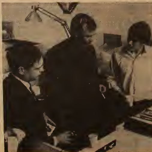
Gerry McMaster, John Andrews and an assistant discuss a floor plan for the Campus Centre.
