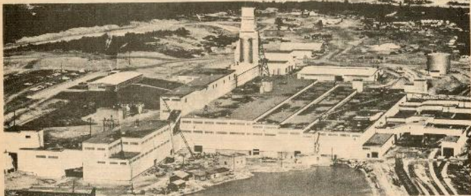
Brunswick Mining & Smelting corporation now owned by Noranda... is one of the world's most expensive smelters.
