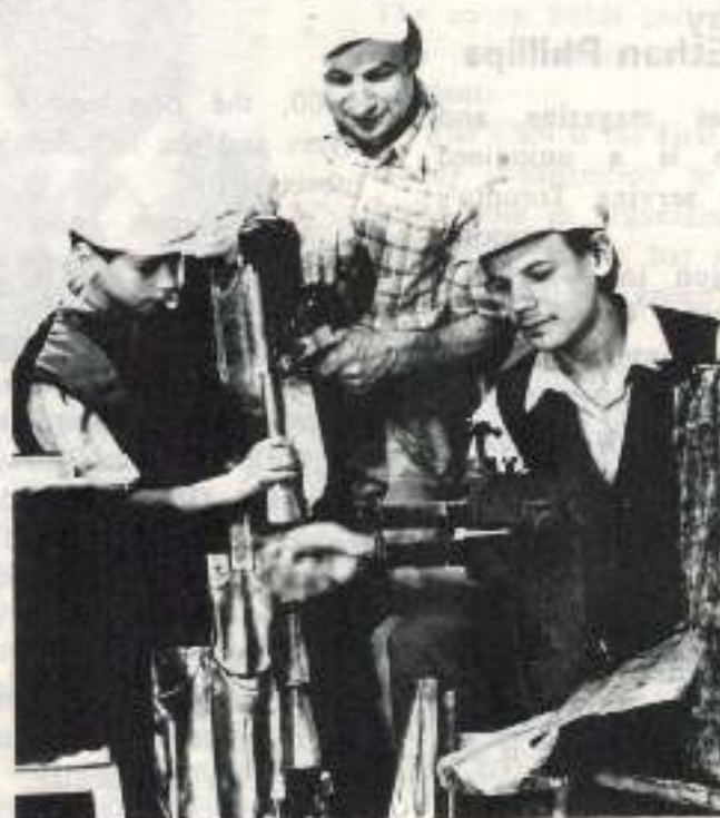
Family co-op to mend gothic roofs in Riga. Anatoly Pashkov and his sons Vitaly and Maxim in their workshop.
