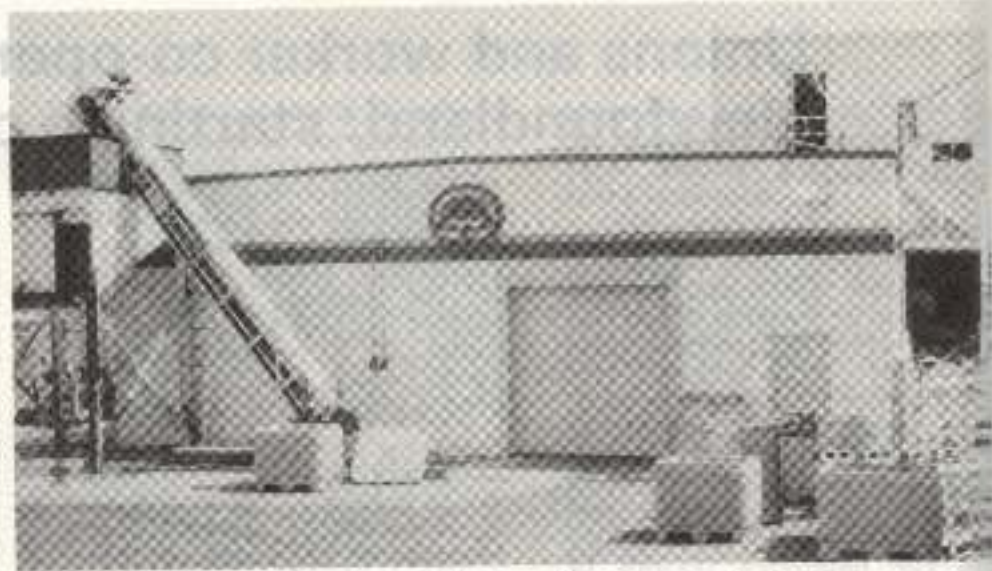
The co-op's fish processing plant in Petty Harbour.
