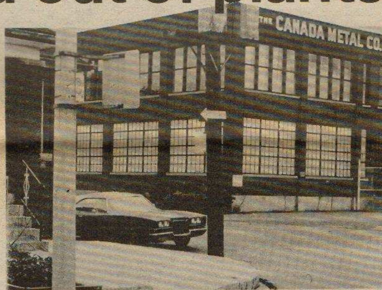
One near neighbour of the Canada Metal plant decided to remove his soil and pollution problem permanently. All that remains is the "Please don't walk on the grass" sign, right next to the "house for sale".
