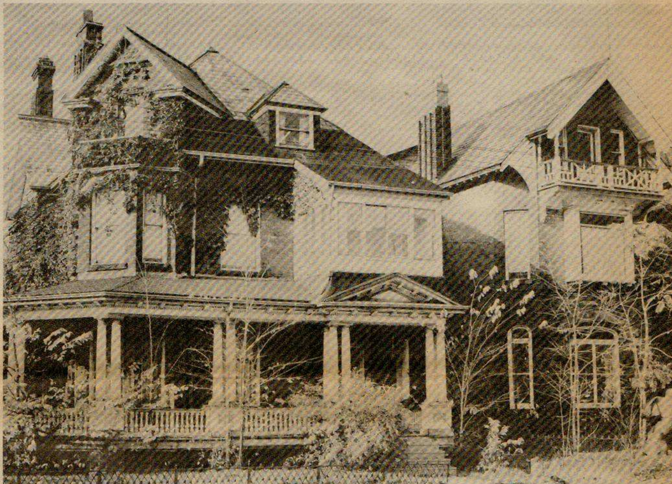
Earlier this year City Council bought out a developer named Amex who planned to wreck several houses in the Annex, among them these two old homes on Huron Street. It cost the City $800,000 to save the houses. The developer, who was generally believed to be an independent company, made an estimated $320,000 on the deal.
