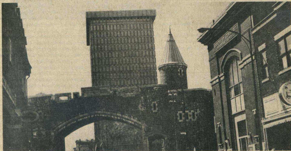
This Quebec City highrise was built by MEPC, one of Britain's largest multinational developers and a main contributor to the current generation of highrises across Canada. Jacob Rothschild, a longtime director of MEPC, resigned last year after a power struggle
